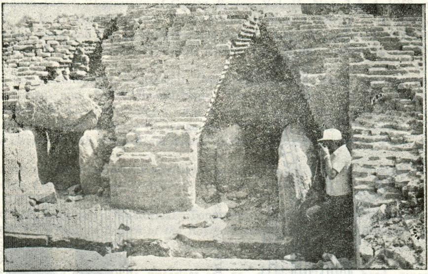
Pl. 1. The inner end of the sluice showing the "trench" in the middle of the cistern and details of the inlets.
